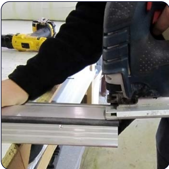
Measure, notch & Cut Threshold to required dimensions.
