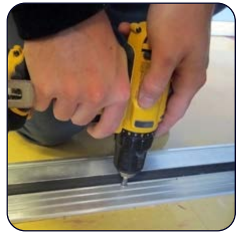
2. Install Threshold.
