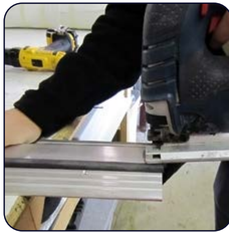
1. Measure & Cut for Threshold.
