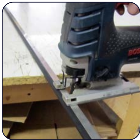
3. Measure & cut door jamb seals.
