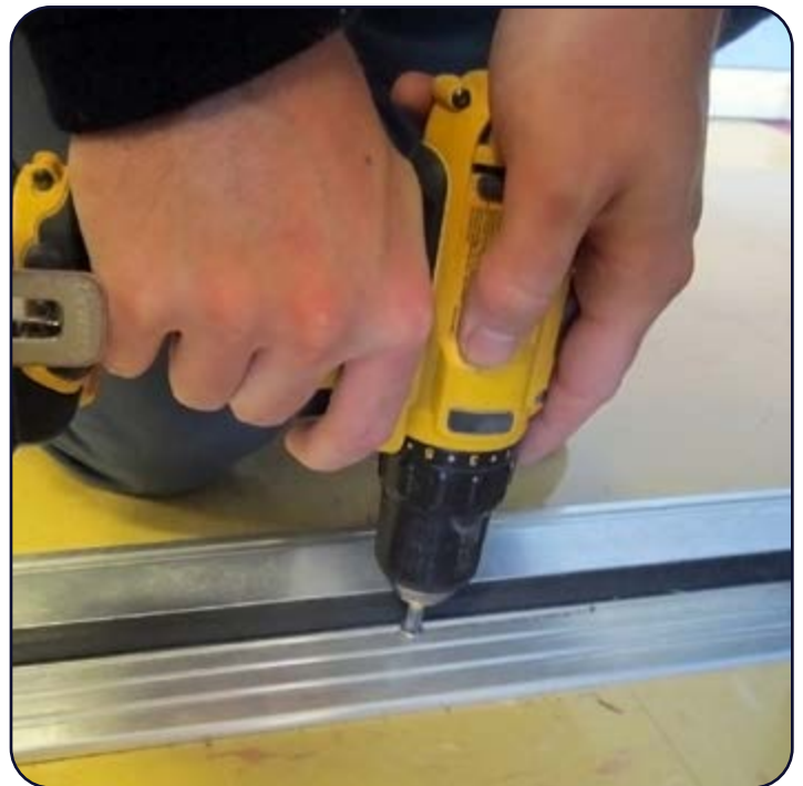
Install Threshold.
