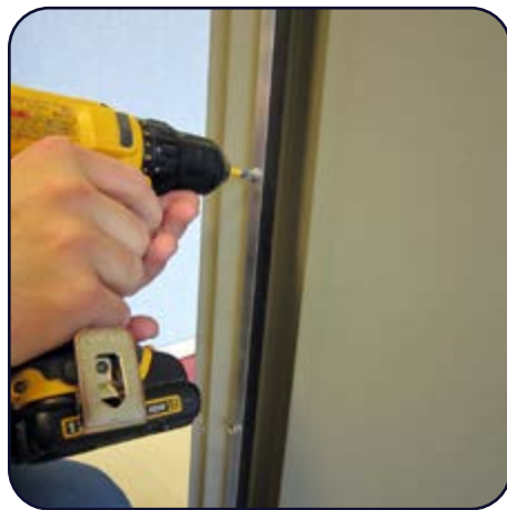
4. Install Jamb Seals to door frame.
