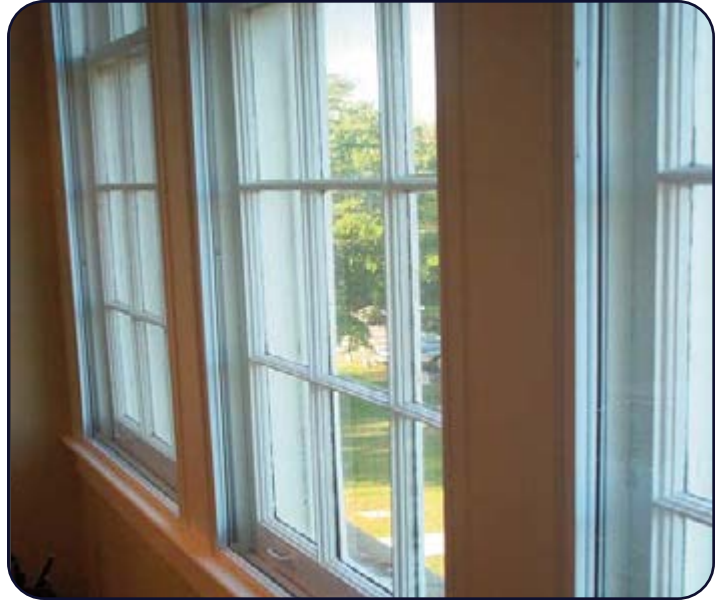
PrivacyShield® Window Seal Kit applied over historic wooden windows at the Mary O'Keefe Cultural Center, Ocean Springs, MS.
